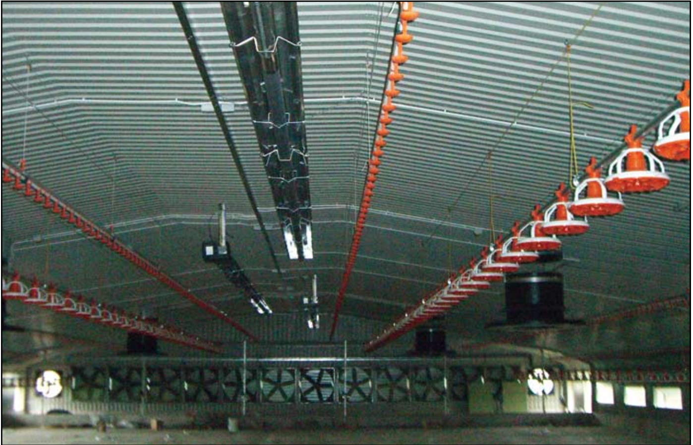
Gas-fired, low-intensity heaters configured for large houses over 75.5' (23 m).
