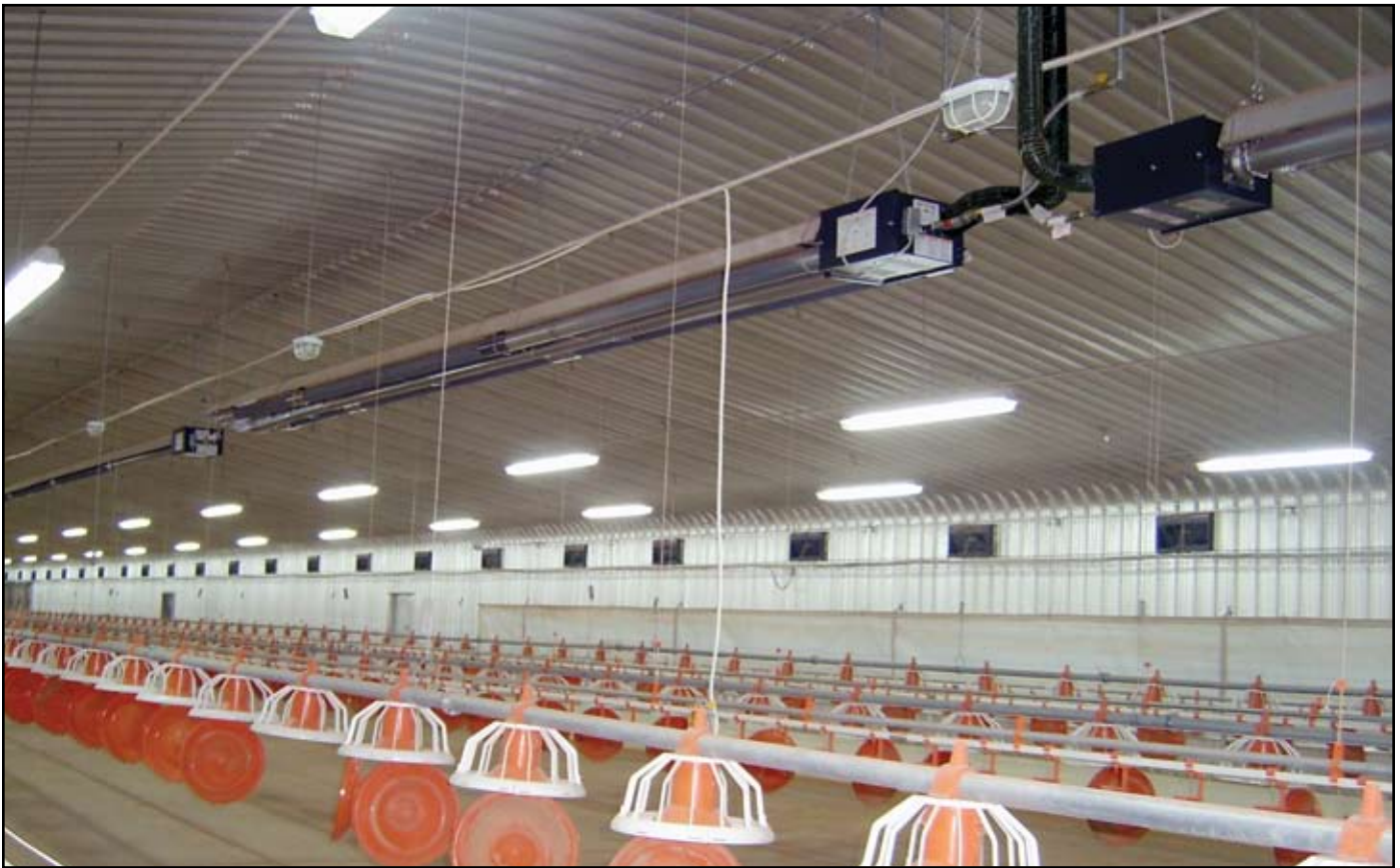
Gas-Fired, Low-Intensity infrared heaters heating a poultry house in the Middle East.
