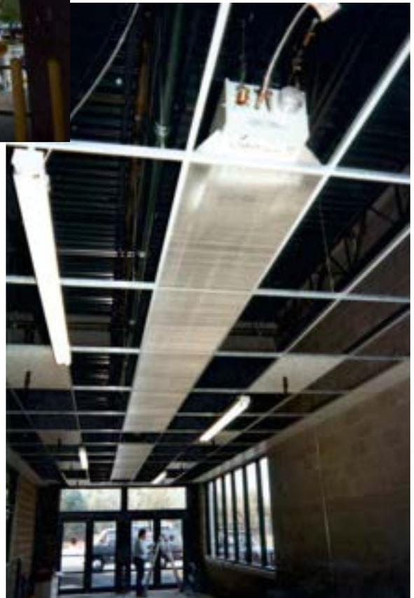
Entrances to stores, passengers terminals and customer pick-up area's can be ideally heated with our gas fired, low intensity infrared heating system mounted over decorative aluminium grille in drop ceilings.
